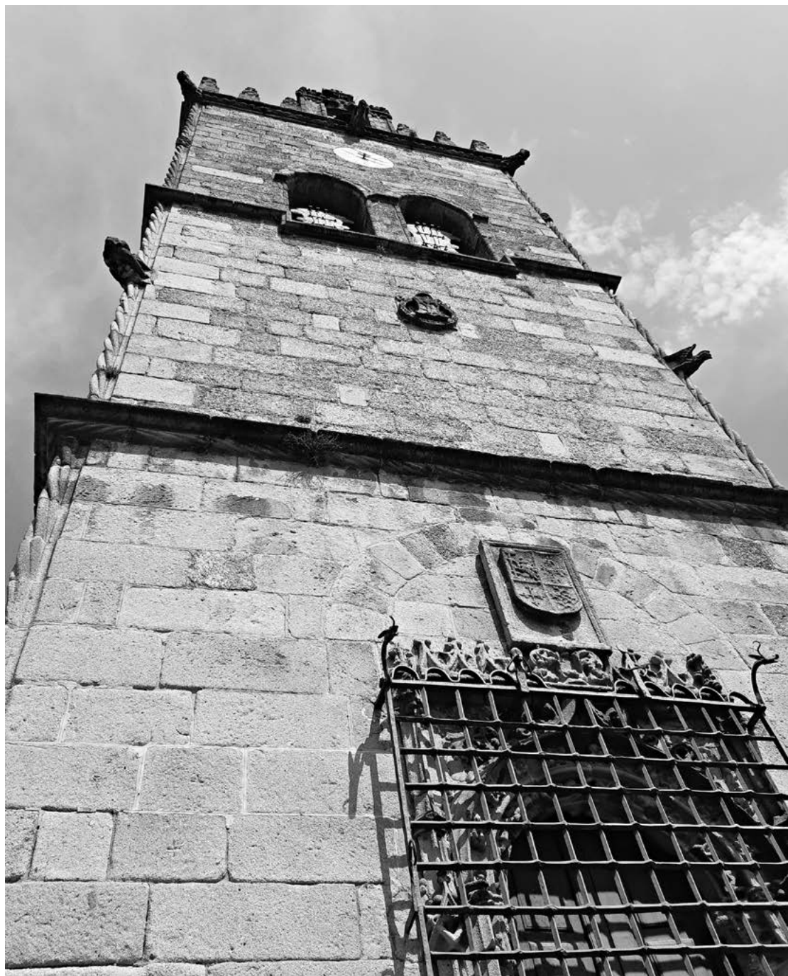
fig. 1. Guimarães, church of Nossa Senhora da Oliveira. Tower of the church (photo Maria José Goulão)
