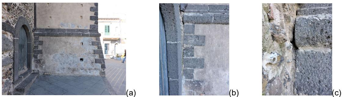
*Figure 3. View of the battered wall at the bottom of the tower on the eastern side (a). The detail of the interface between the quoins of the battered wall of the tower and the surface of the wall of the church (b) could demonstrate the absence of structural connection. It is clearer in the detail picture of a single stone block of the lower cornice (c).*
