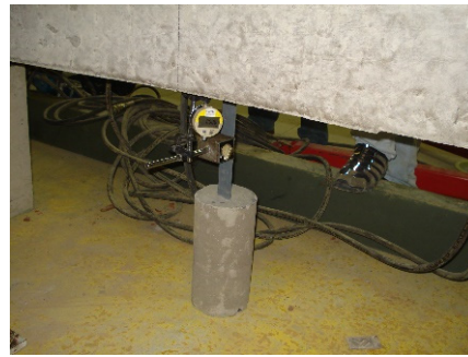
(c) Detail of instrumentation
