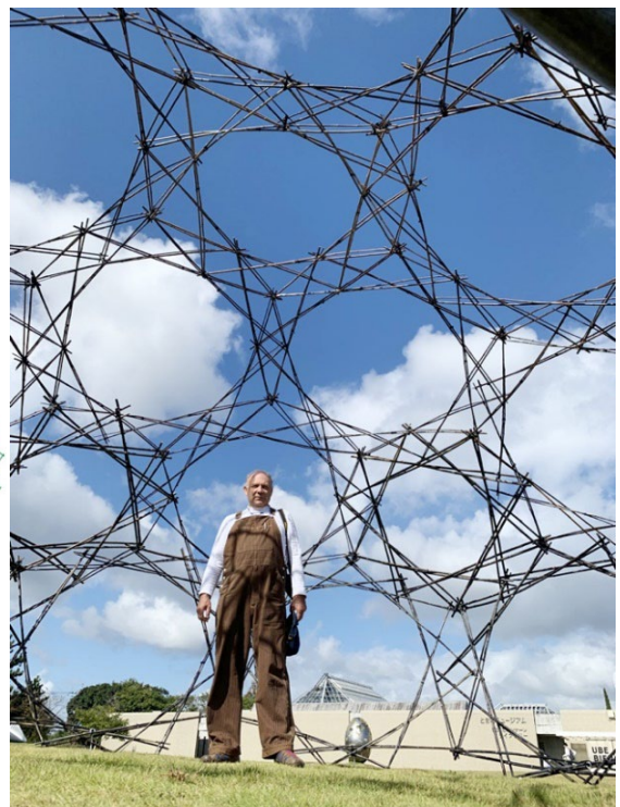
Figure 7 On the left the assembly-diagram of a fullerene C80 bamboo dome made from 6 decagonal and 20 dodecagonal stars. Note that all the bamboo-stars are double layered and made from 600 bamboo struts of 2-m. Assembled in half a day to a dome with a diameter of 8m and a height of 5m and a weight of 100 Kg. Ube Sculpture Biennale Japan 2021.
