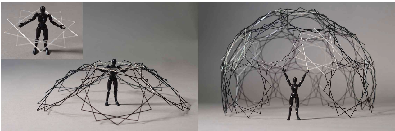
Figure 9 Left side: Starting with the top centre decagonal star, where on its edges five dodecagonal stars are attached to. Right side: The 5/8 dome is built from the top downwards and there is no need for a crane or scaffolding! The row of the 10 dodecagonal stars is standing all on the ground and one is left empty for the entrance. Model size M = 1 : 200 .
