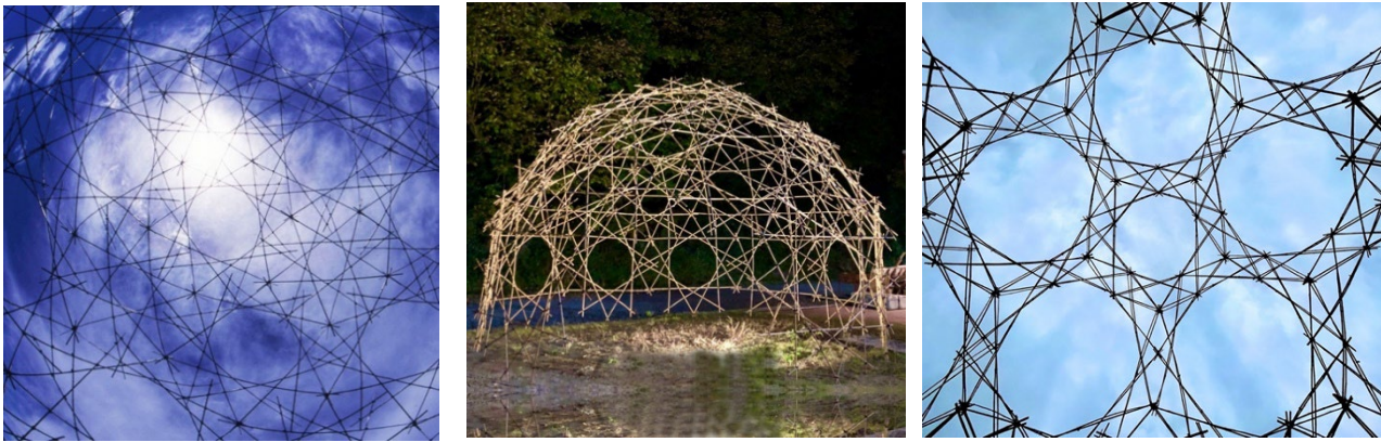
Figure 8 Fisheye view of a fullerene C60 dome. Snow crystal like fullerene C80 dome. Filigree like a giant Radiolaria; the top section of a fullerene C80 bamboo dome using the new weaving-method with big openings to see the open sky.
