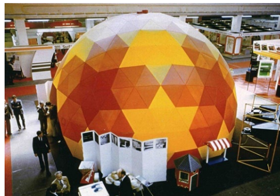
Figure 1 A 6-frequency icosahedral paper dome designed by the author for Swiss Pack Expo Basel 1971. Note that the distance between two centres of the pentagonal stars is divided into 6 edges i.e., 6-frequency. Diameter 8m, height 5m.
