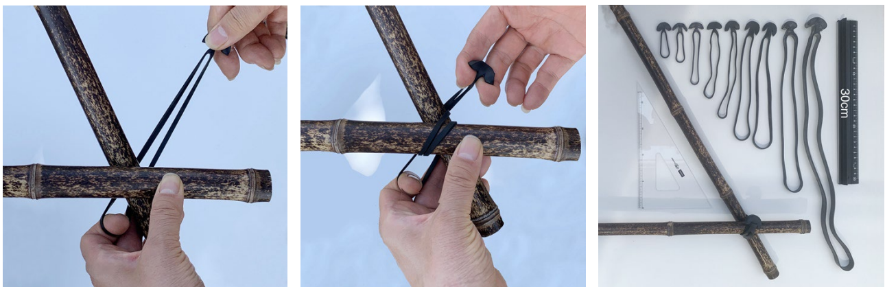
Figure 4 Lashing technique of the bamboo struts using rubber connectors. For a 5/8 dome we need 800 pcs. connectors. The mushroom-like rubber head is pulled and wrapped twice around the bamboo, then secured by hooking into the tale.
