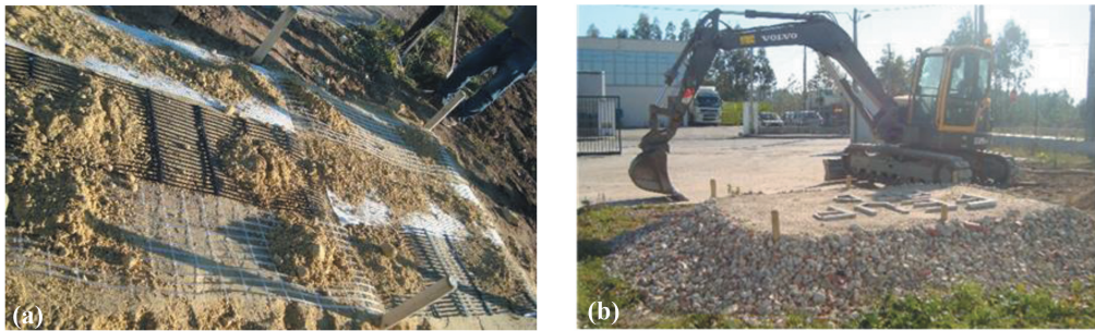
Figure 3. Trial embankment: (a) placement and arrangement of geosynthetics; (b) finished embankment with lateral protection with coarse aggregates.
