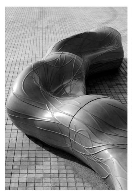
11.08. XURRET's organic concrete: the complex curvature and intricate surface veins perfectly match at the contact sections.
